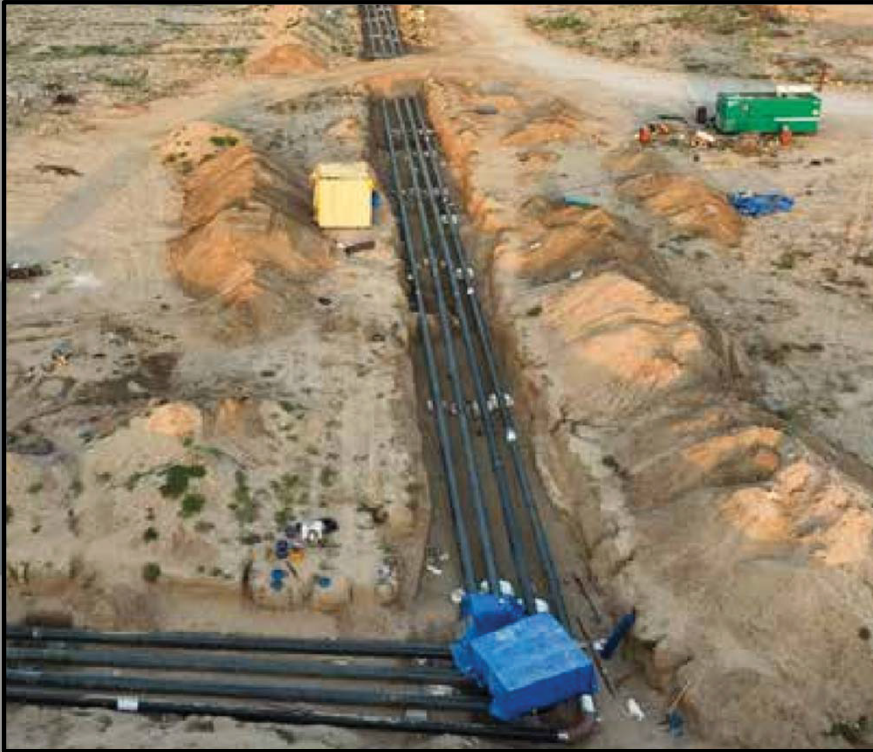
PIPELINE & PIPING PROJECT SOMGAS, BERBERA, SOMALILAND
