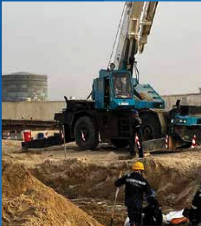
35 TON FOUR WHEEL CRANE
