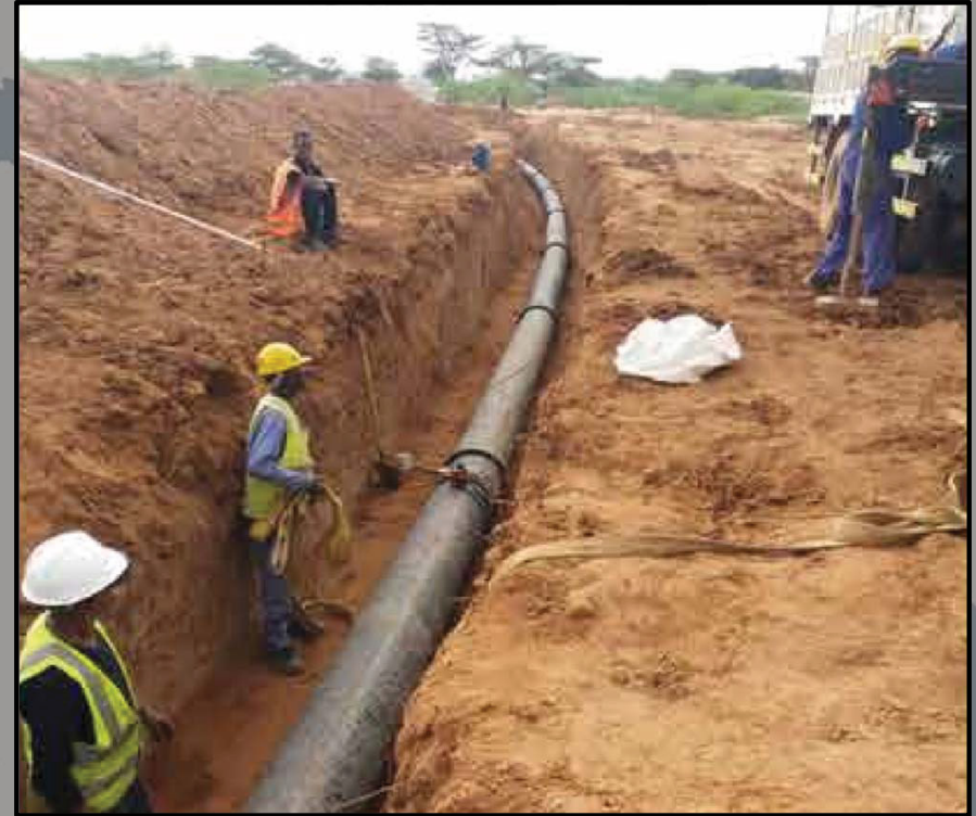
PIPELINE & PIPING PROJECT SOMALILAND DEVELOPMENT FUNDS, GEED DEEBLE, SOMALILAND
