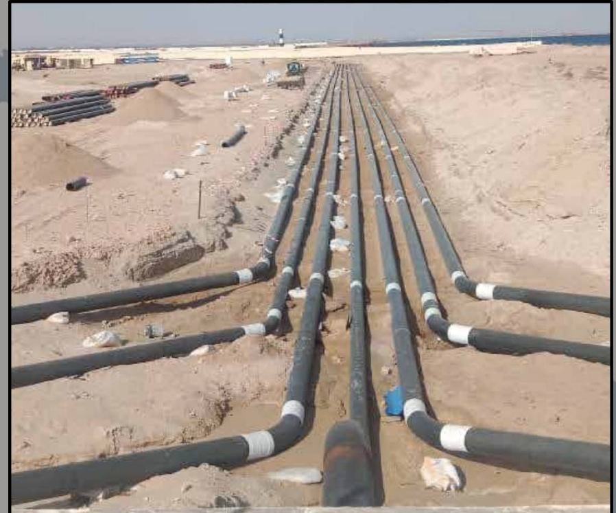
PIPELINE & PIPING PROJECT ARDMORE ONSHORE LINES, BERBERA, SOMALILAND
