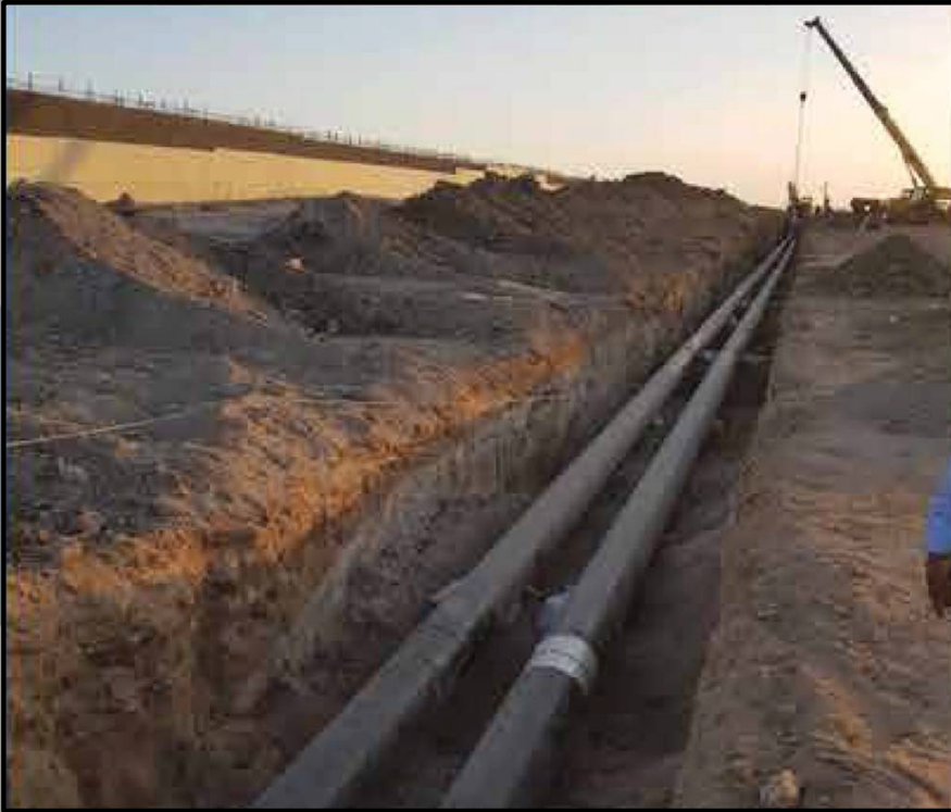
PIPELINE & PIPING PROJECT DAHABSHIIL OIL STORAGE TERMINAL, BERBERA, SOMALILAND
