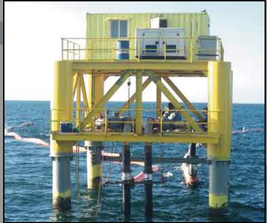
MARINE & JETTY PROJECT DOST, BERBERA, SOMALILAND
