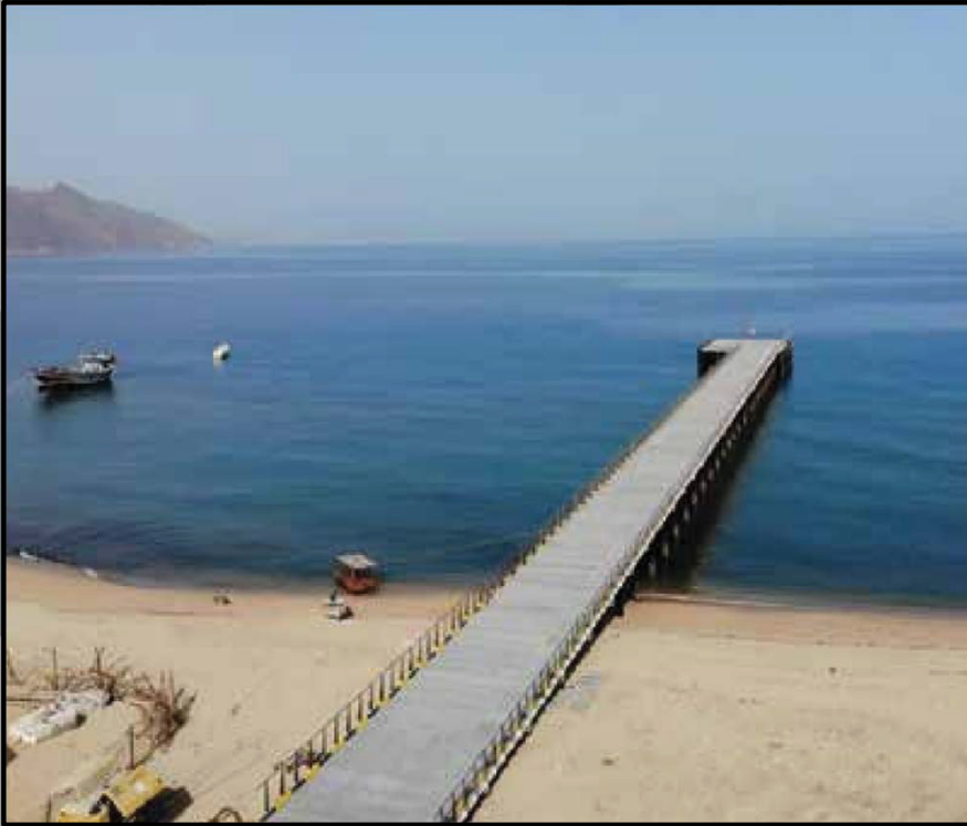
MARINE & JETTY PROJECT MINISTRY OF FISHERY MAYDH, SOMALILAND
