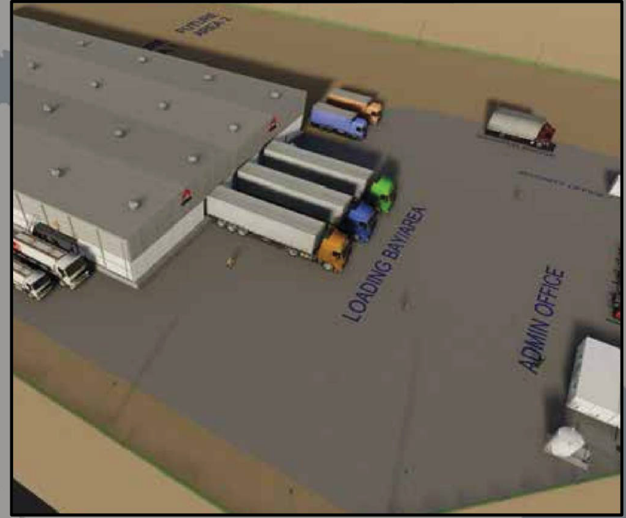
INDUSTRIAL WAREHOUSES PROJECT IFFCO, SAHEL BERBERA, SOMALILAND
