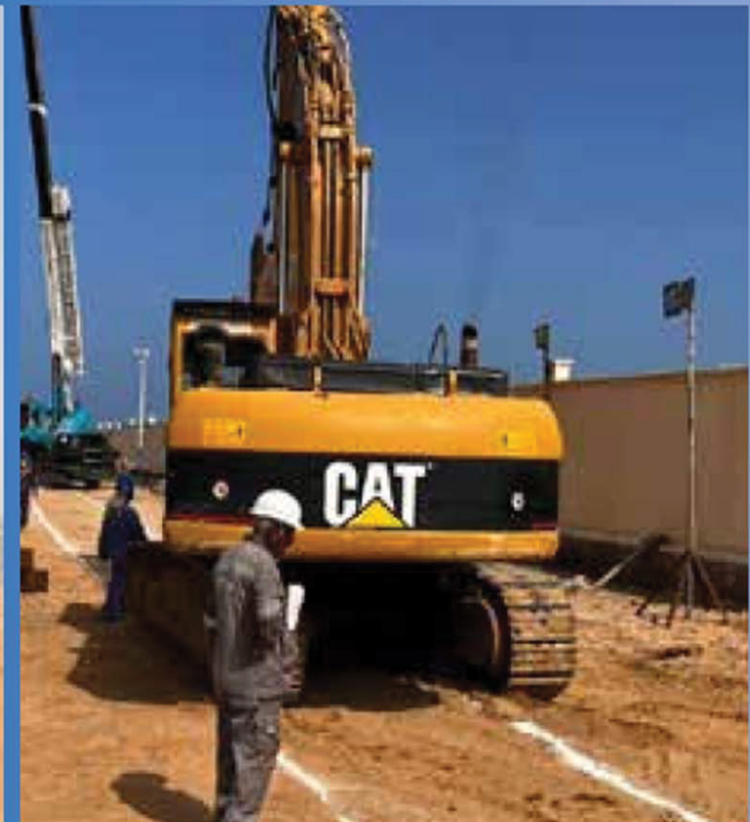
330 CL EXCAVATOR CAT
